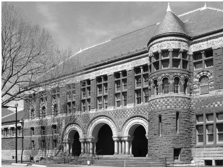
Austin Hall, a classroom building of the Harvard Law School.
